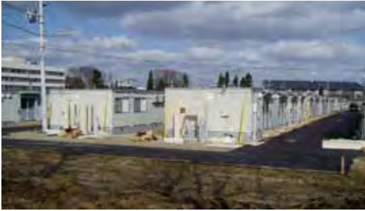
▶ Temporary housings in Nigata
